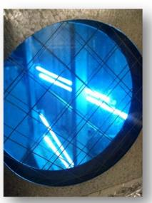
A properly sized and installed set of lamps will noticeably clean a coil in about 30 days with continued improvements up to one year later on severely clogged coils. The UV-C fixtures can be installed in about two hours at an installed cost (materials and labor) of roughly \$0.15 or less per CFM of airflow capacity. For the Kentucky Medical
